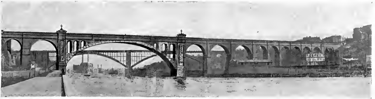
ACCORDING TO THE PLAN SUGGESTED BY THE ABOVE DRAWING FOUR PIERS WOULD BE REMOVED AND THE RIVER SPANNED BY A SINGLE MASONRY ARCH
